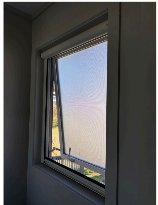
Fitted to the inside of an awning window (our standard fit) - Lake Taupō.
